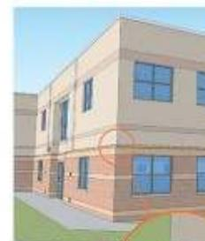
Existing unflashed soldier course brick replaced with three courses of matching level brick caprow with flashing (waterproofing tucked under existing EIFS system).
