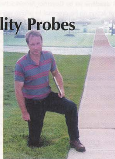
Engineer Michael Pierce stands knee-deep in a sinkhole in this photo, which ran in a number of newspapers after it was displayed at hearings held by New Jersey state investigators. The cause was traced to an unconnected drain pipe joint, which Pierce believes was overlooked by town inspectors.
