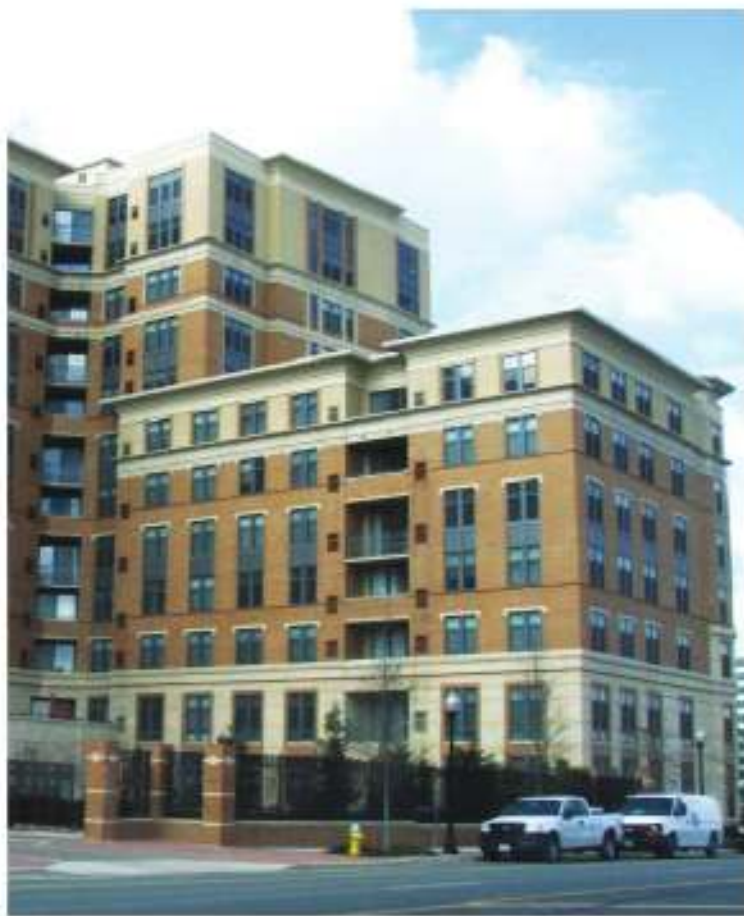
Approximately 1670 m 2 (18,000 sf) of EIFS was used at Camden Potomac Yard, a luxury, multi-family, high-rise apartment building in Arlington, Virginia. Work involved finishing the cornices around the top of the building, as well as its ceiling.
