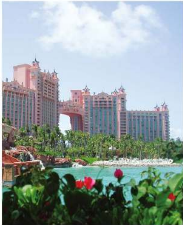
The EIFS walls used on this hotel and casino can withstand 250-km/h (155-mph) hurricane winds.
